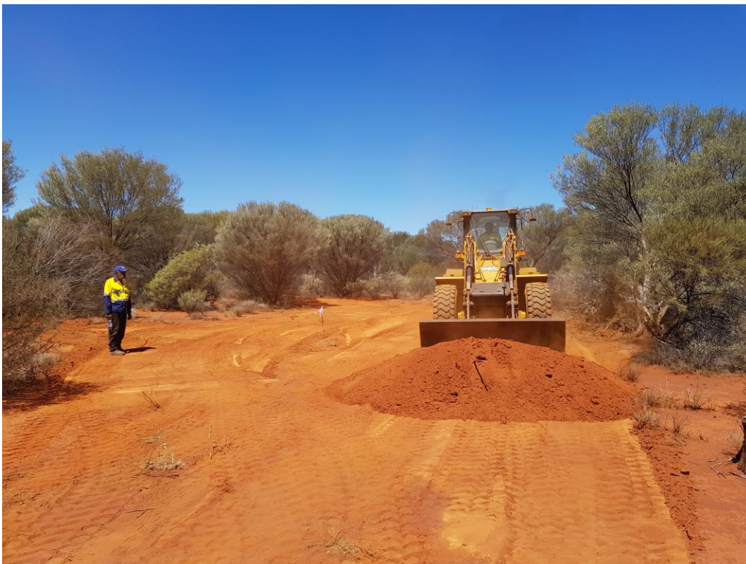
Figure 9 - Access and drill pad preparations - March 2018
